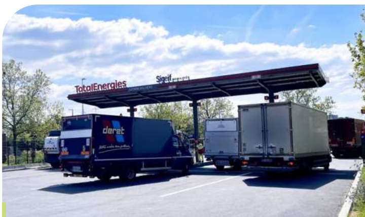
Station GNV-Bio-GNV à Gennevilliers.
